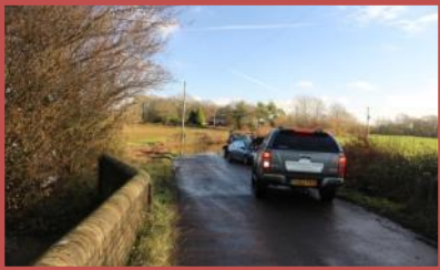
Flooding at Flash Bridge, taken 02/01/2014
