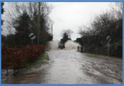
Flooding at Alfold Road exit, taken 24/12/2013
