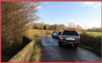
Flooding at Flash Bridge, taken 02/01/2014
